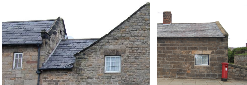
(1) Parapet detail to Lilac Cottage (2) simple stone coped gables seen extensively
