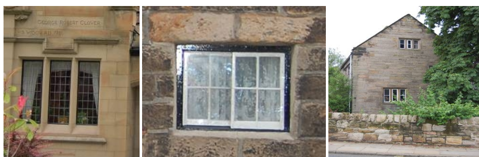
Windows in the conservation area (1) leded lights (2) sliding casement windows(3) stone mullioned, window casements
