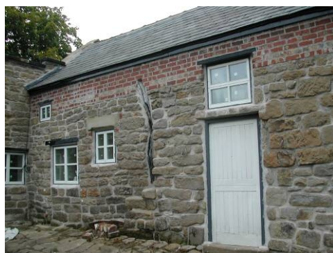
Barn to Stone Farm; stone with cruck frame evidence. Brickwork possibly resulting from lowering the roof pitch following replacement of thatch by slate.
