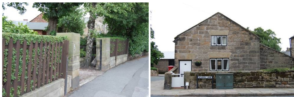
(Left) Gate posts to Clover Cottages; (Right) Boundary wall to Stone Farm
